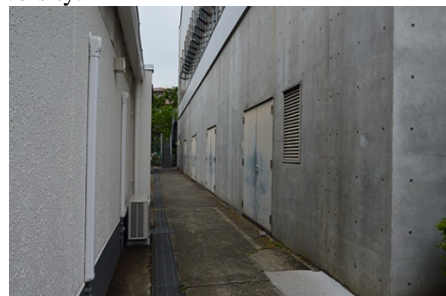
Fig7. Building No.14 of the Setagaya Campus in Tokyo City University
